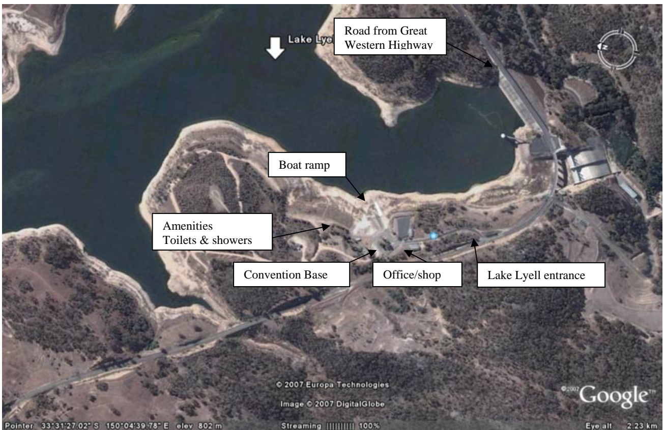
Lake Lyell – indicating Dam wall, entrance area, office/shop, convention base, amenities, concrete boat ramp.
